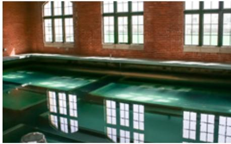
Water is then passed through a sand and gravel filter bed, removing any remaining suspended matter.
