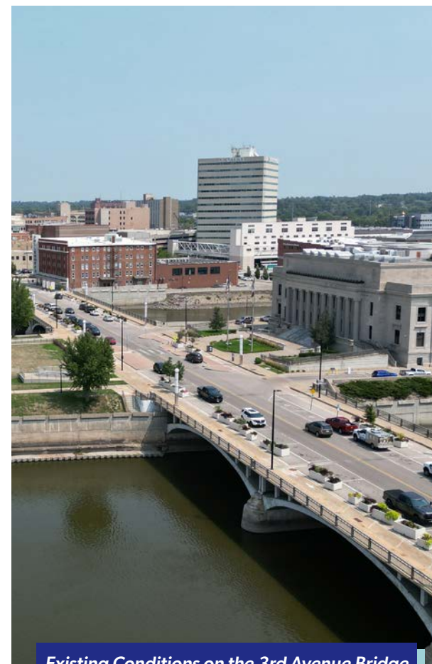
Existing Conditions on the 3rd Avenue Bridge
